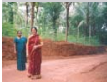
Field workers in the Road constructed in Punnaikunnam Ward
