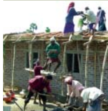
Construction of a house using cost-effective technology, Vadakarapathy
