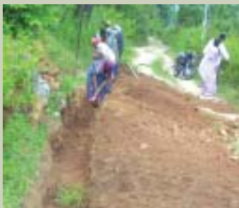
Renovation of earthen channels under NREGS, Vadakarapathy
