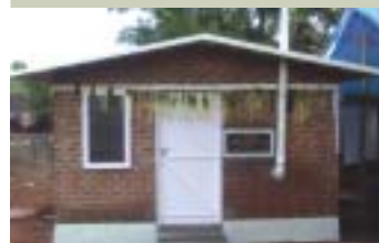
The first house built for destitutes using cost effective technologies in Eruthenpathy
