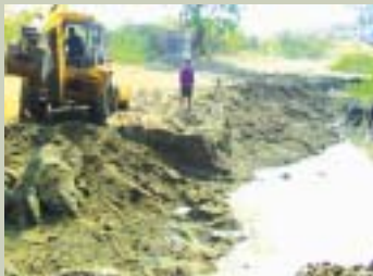
Pond renovation work under progress at Chinnari in Vadakarapathy
