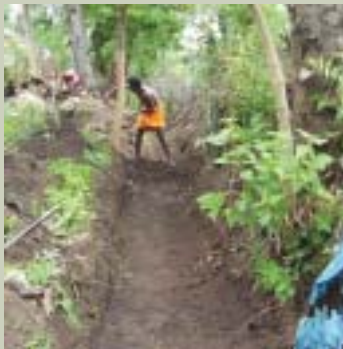
Renovation of earthen channels by NHG, Vadakarapathy
