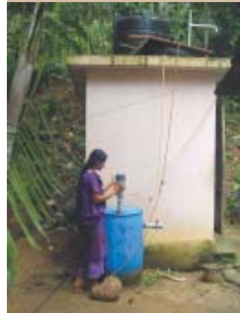
Sustainable settlement model- Domestic bio-gas plant
